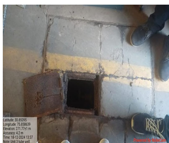
View of Bore well @ unit Location 3
