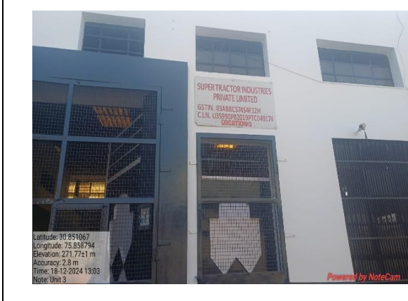
View of Gate at Location-3 unit
